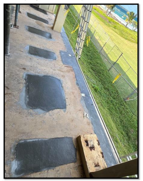
Patched spall repair along lanai slider
